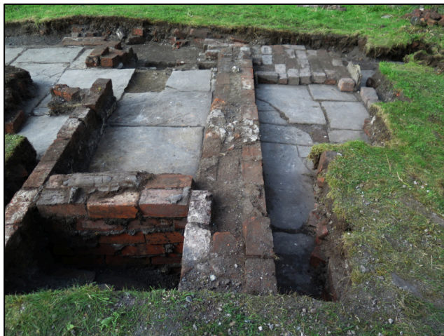
Fig.5: 2021 photo showing internal brickwork and wider external wall.
