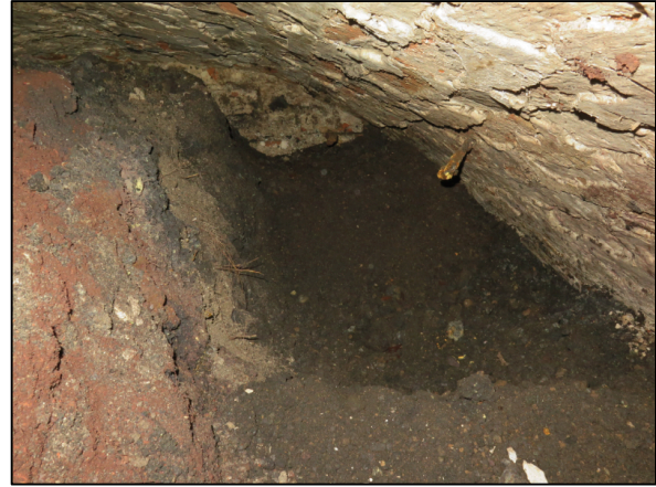
Fig.10b: Inside of Vaulted Cellar with white washed walls
