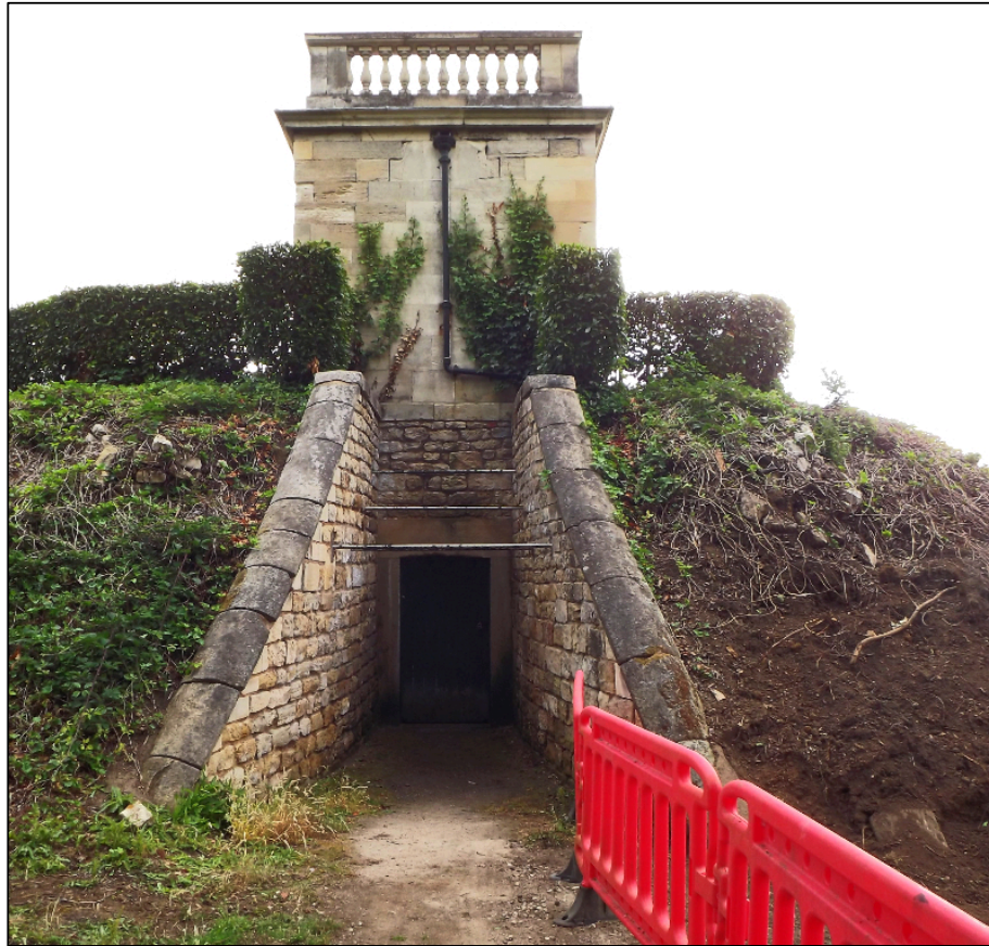
Fig 4. West side of Summer House mound with entrance to ice house, note collapsed stonework on right hand side © J Buglass
