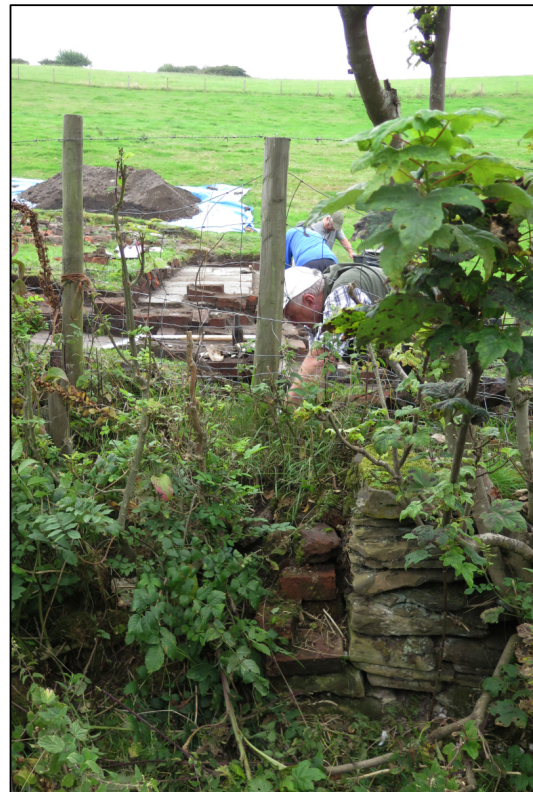
Fig.4: View from the road, showing transition from stone wall to brick work of possible loading platform.
