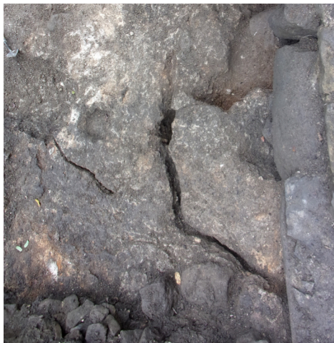
Fig.4 : Evidence for subsidence of the east cross wing
