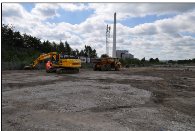
Fig. 2: A general view across the site prior to excavation
