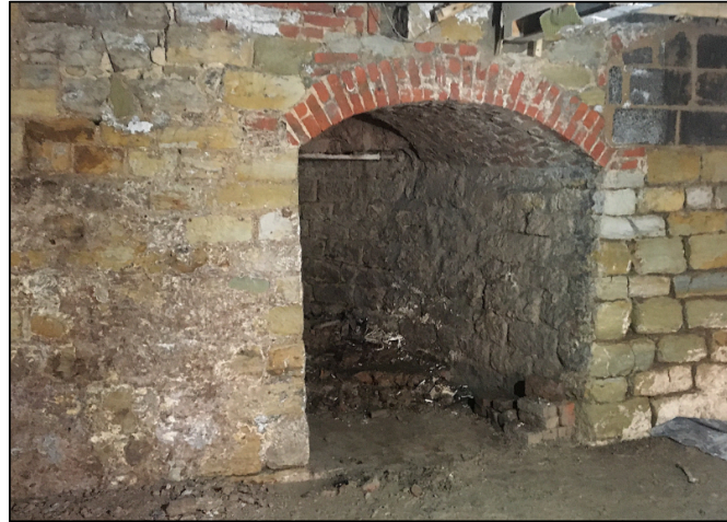
Fig. 4: View of the arched opening of the former lime kiln.
